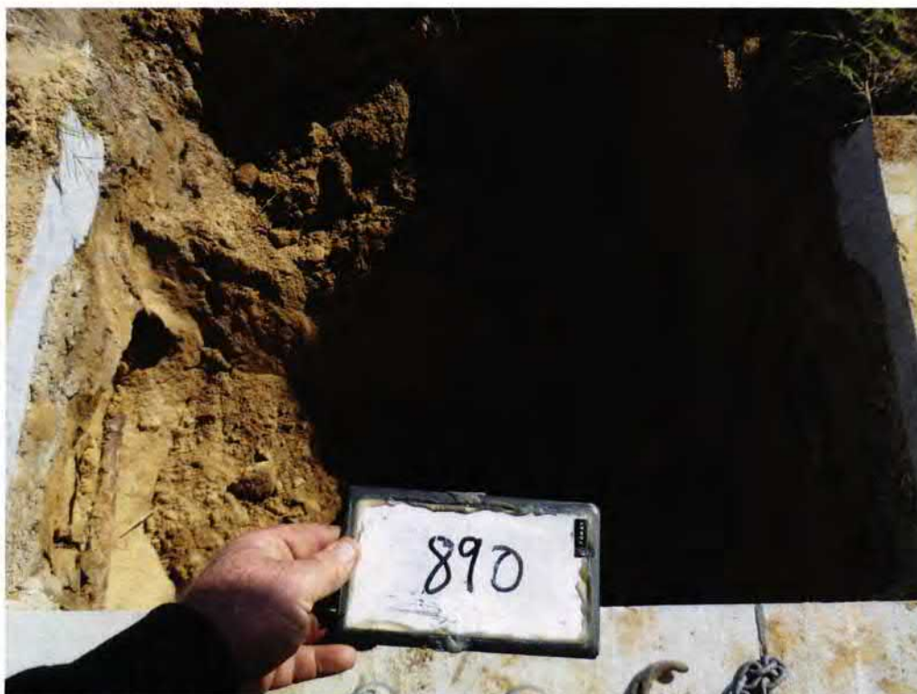
Picture 2: UST 890Cobia excavation.
